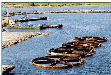
August 1999 - Brent Spar complete the quay foundations
