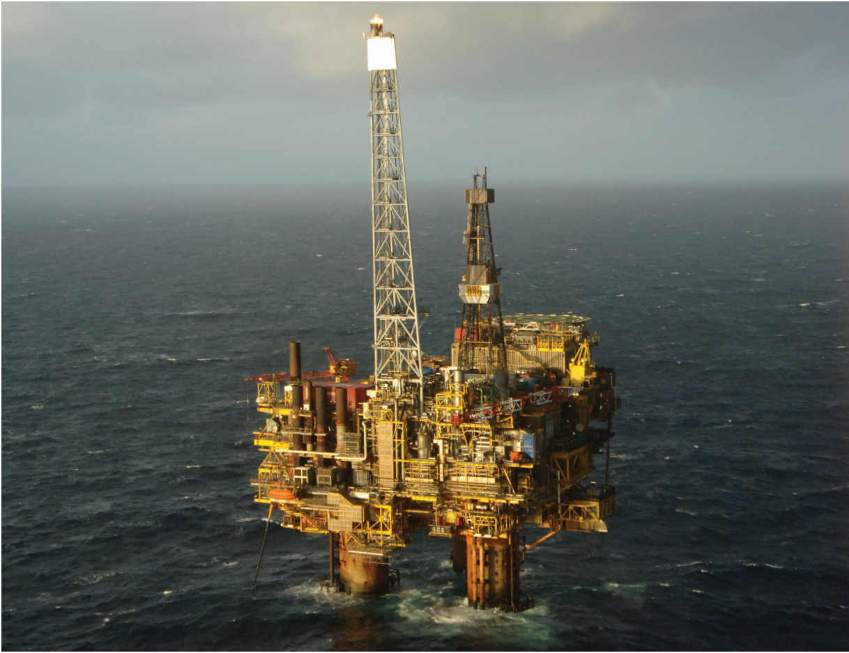
Brent Bravo production platform is a concrete gravity structure with three legs
